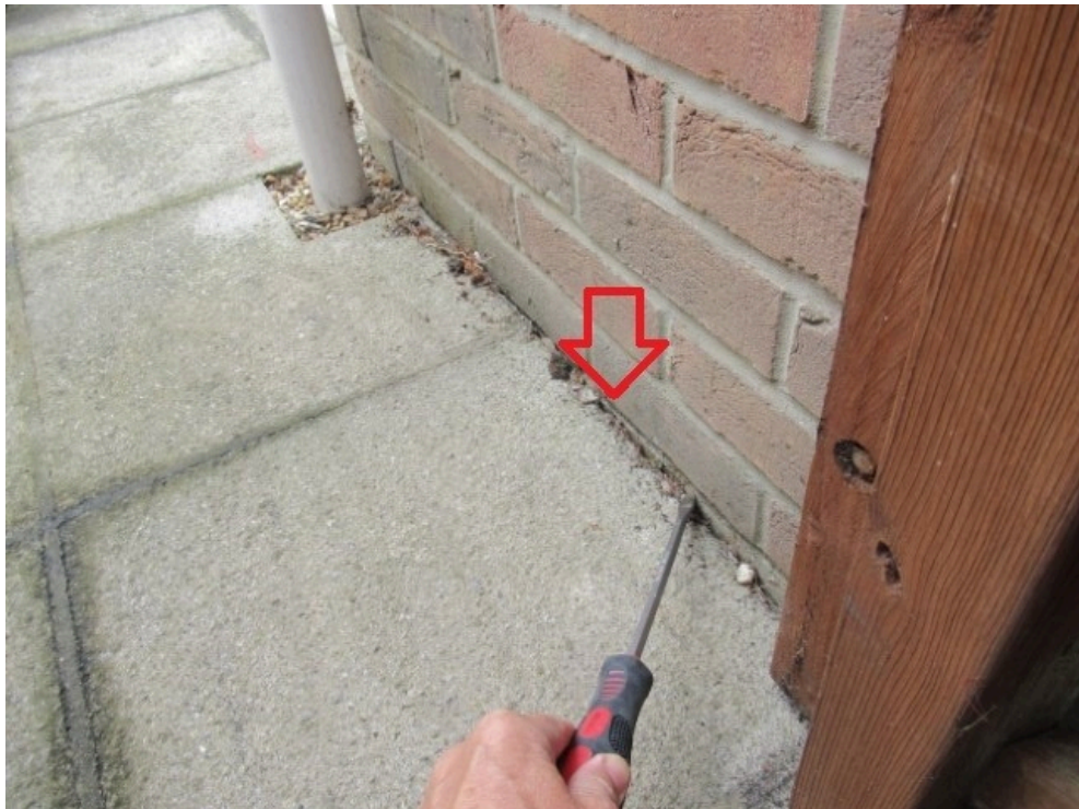
Level of damp proof course on the right side adjacent to the porch
