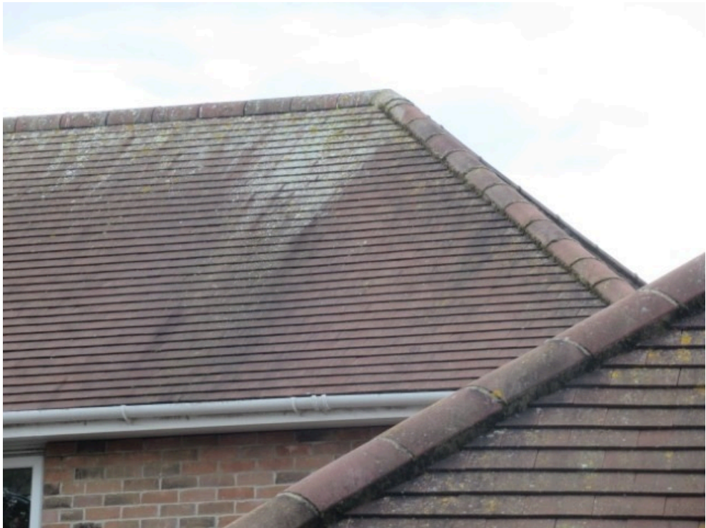
Right side roof pitch
