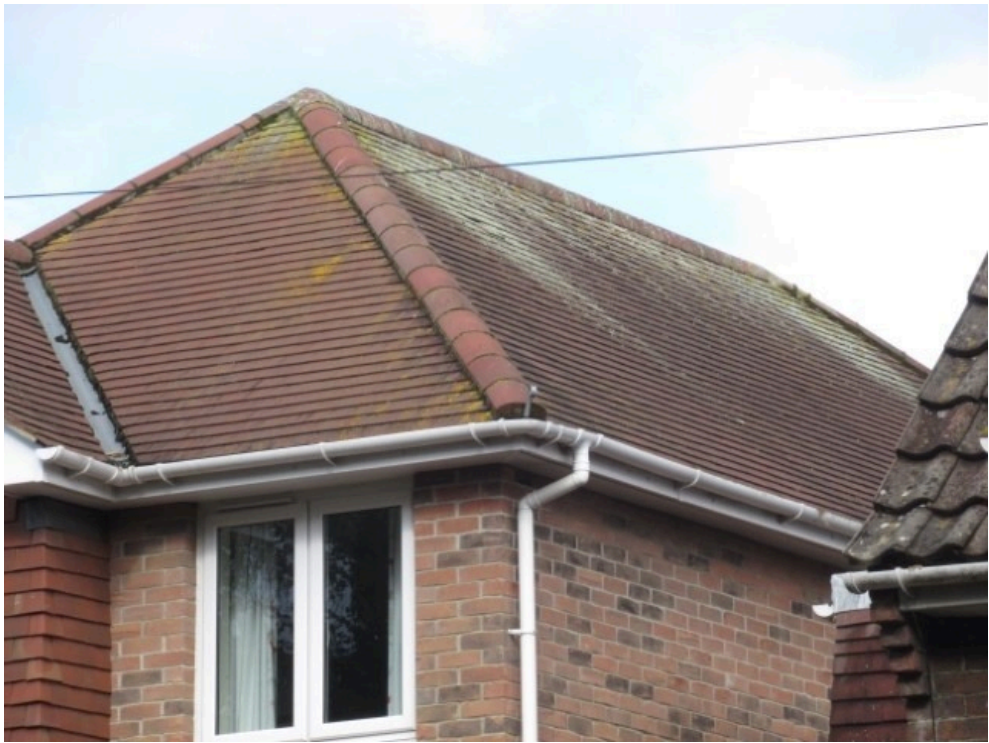
Front and right side roof pitches
