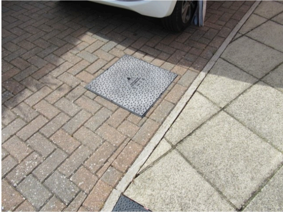
Inspection chamber in the drive
