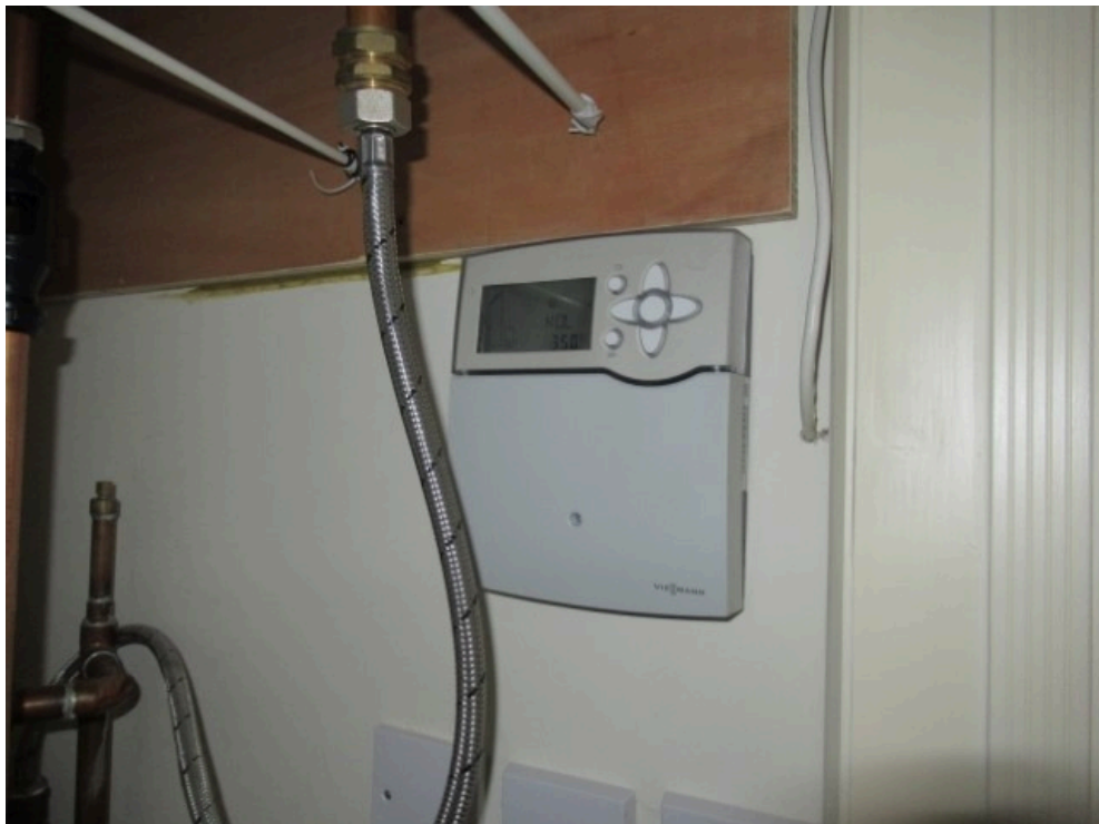
Control panel for the solar water heating panels
