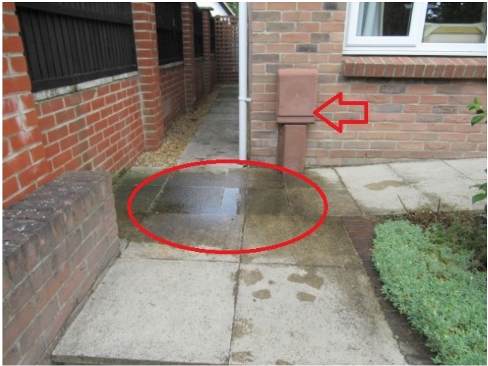
Wet path adjacent to water meter housing
