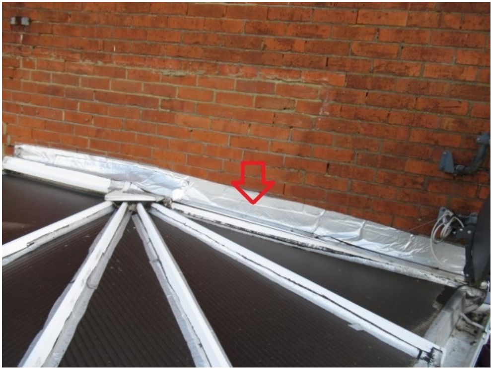
Flashband flashing
