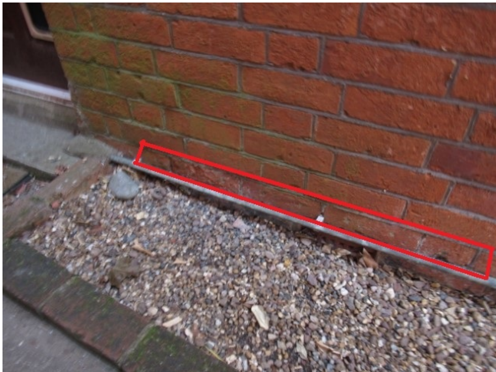
Injected DPC holes on the left side wall
