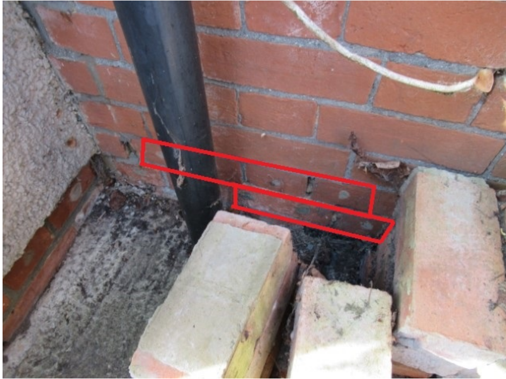
Double layer of injected DPC to the right of the bay at the front
