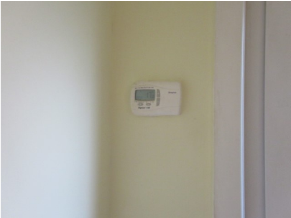
Combined programmer and thermostat
