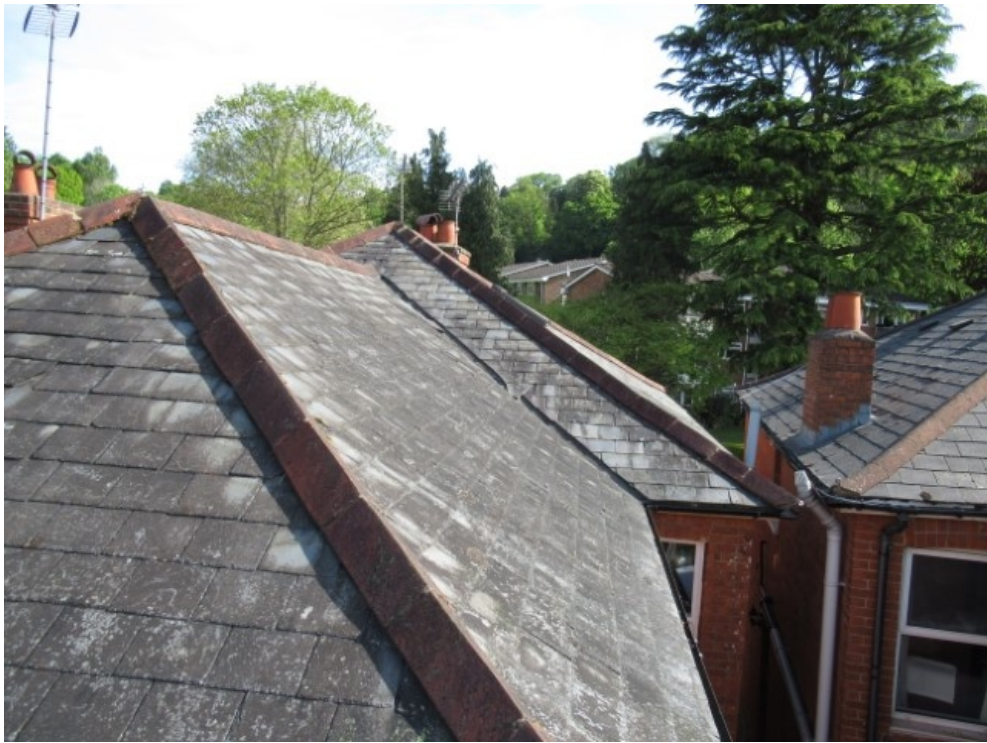
View of rear addition roof
