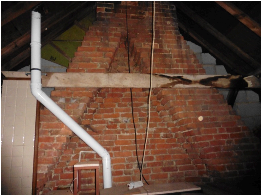
Front and rear chimney breasts in the roof space
