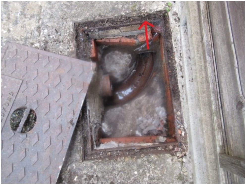
Inspection chamber to the left side rear with the house to the left of the picture
