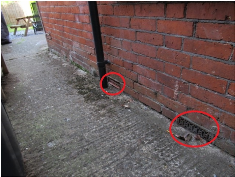
Air bricks on the left side wall
